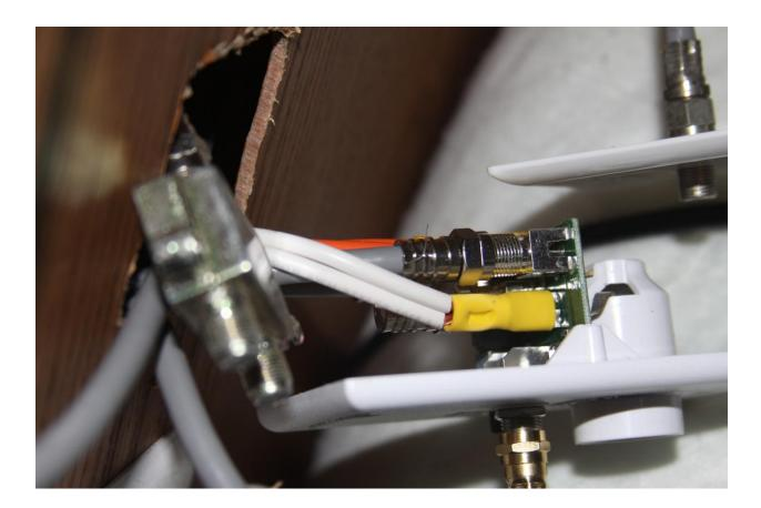
The cable for the park cable television has pulled out and dropped somewhere in the wall. You can see the screw on connector just below the two white wires. So this is why the park cable did not show any continuity.
