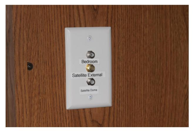
The center connection has been installed, the plate mounted back on the wall, and each connection is labelled for future reference. Prior to installing the plate, I tested the connection to the external satellite input to make sure that the cable was working. It was so this is the end result. Now I can use the external connection with the ground dish.
