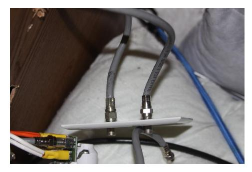
This is a picture of the splitter once the cables to the external connection that says "Wired for a Winegard Digital Satellite System and the roof dome have been removed.
