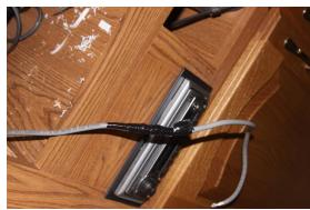
you need to remove the tape for some reason. Next we feed the cable back through the hole in the wall and connect it to the Winegard park antenna connection. I had to take the power lead off and one of the other cables in order to have enough room to work. The assembly was then tested to make sure that the cable connections were good. I used the same device to short the center lead to the outside screw on connector. Reconnect the power
